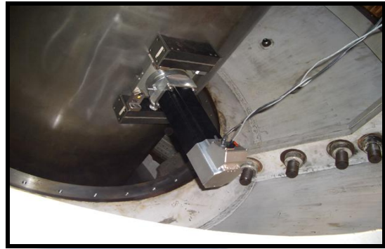
Sancheong pumping-up power plant
