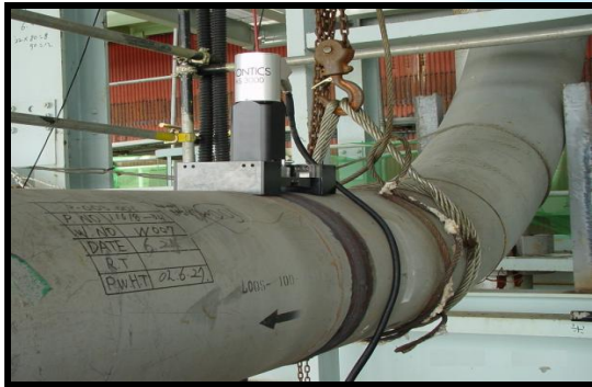
Youngheung thermoelectric power plant
