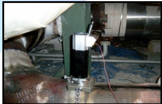
Ulsan thermoelectric power plant
